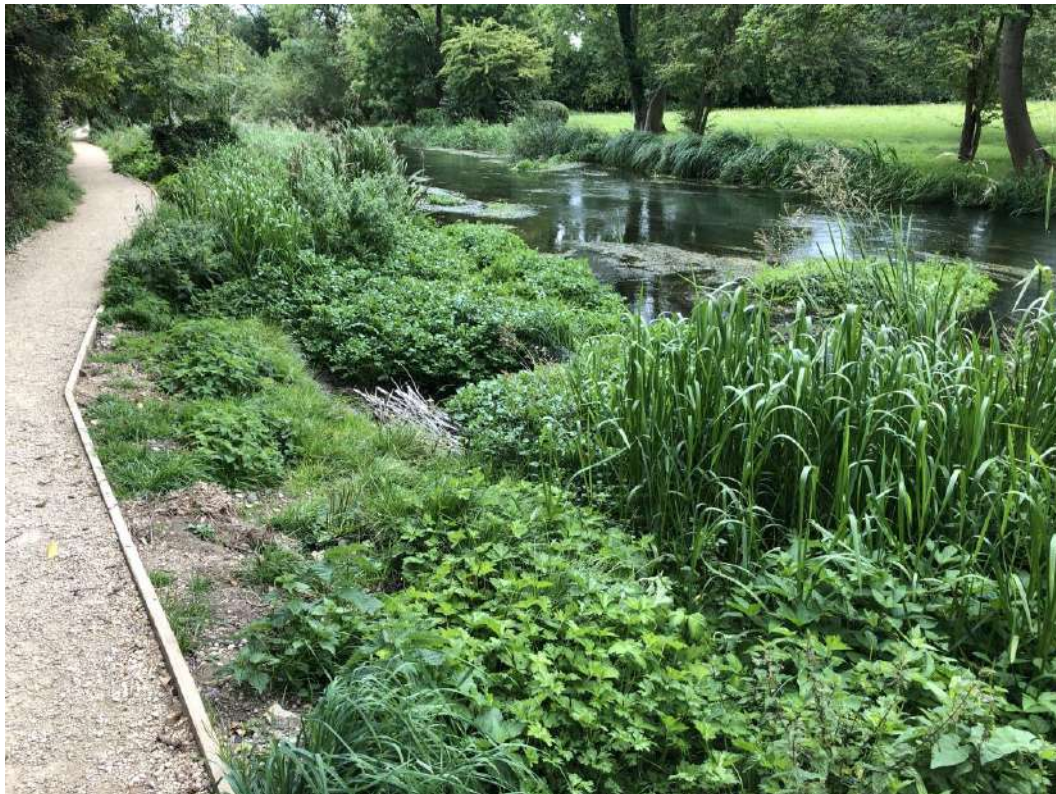
Coir fibre rolls installed in Section 4/5; water voles present
