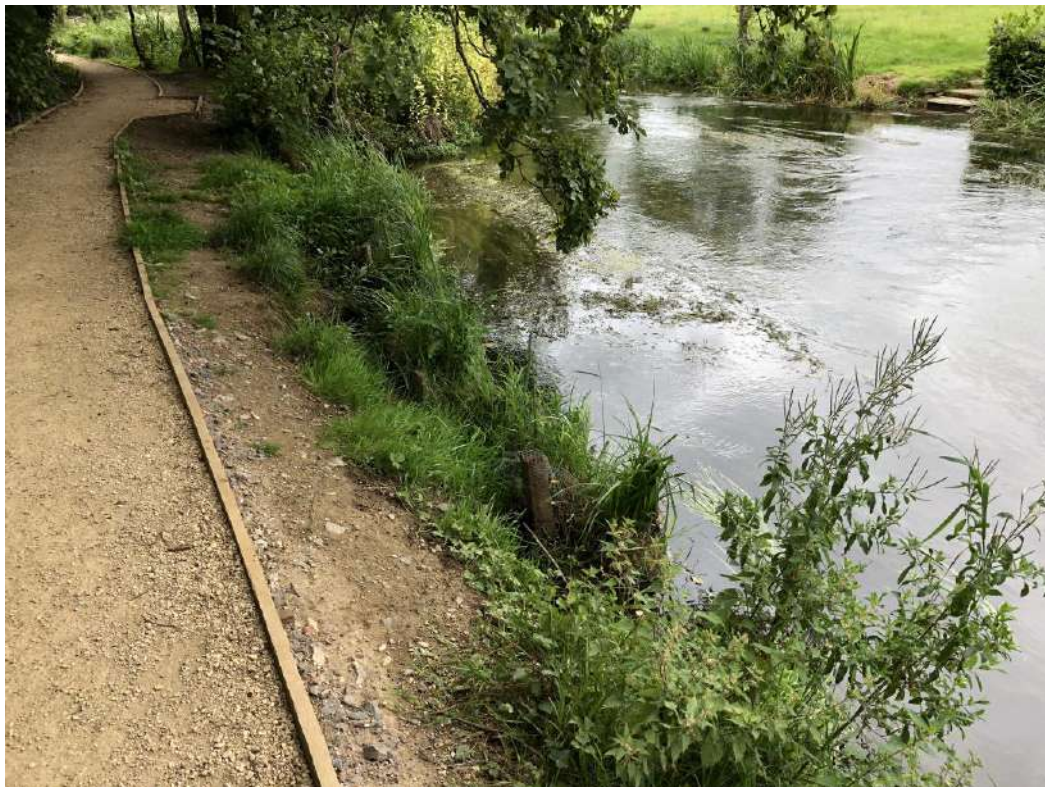
Coir fibre rolls installed in Section 3 where displacement took place; vegetation still establishing
